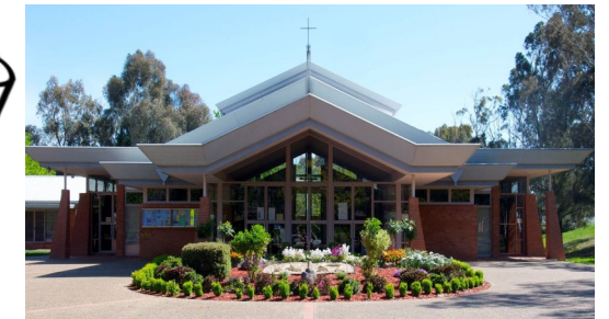
St Michael's Church Tyrrell Cct Kaleen
